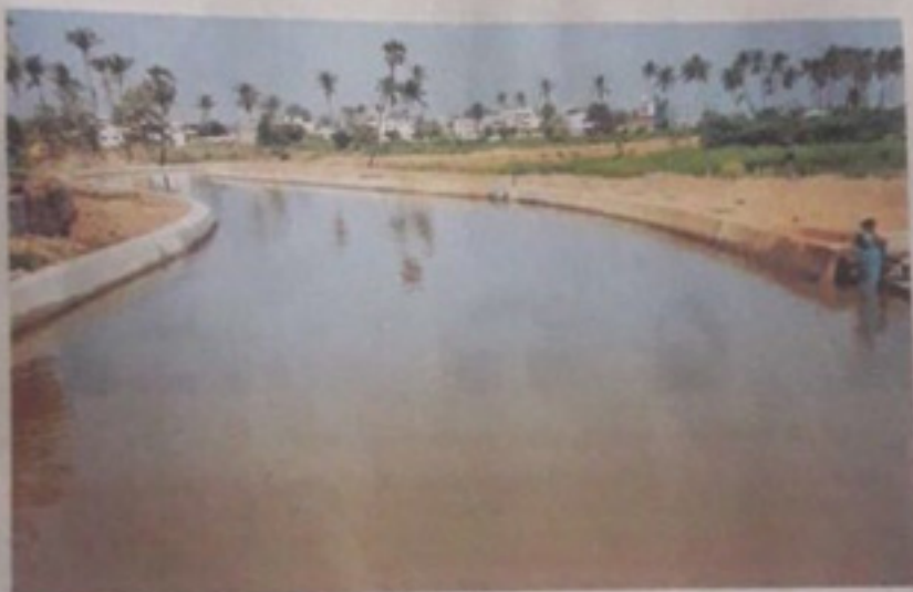
The Kalingarayan Canal was built nearly 700 years ago
